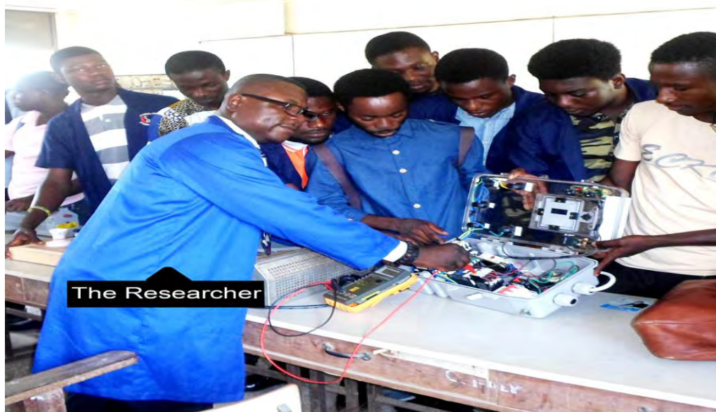
Figure 4.5: The researcher assisting students in construction of star/delta starter for corn mill motor.
