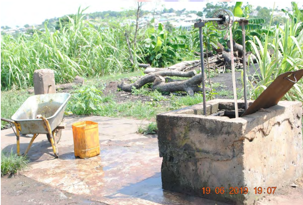
The supporting poor conditioned well.
