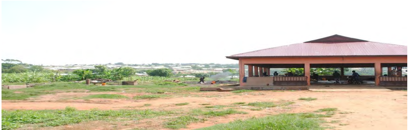
Plate 3.1: The structure of the slaughterhouse in Kintampo North Municipal.
