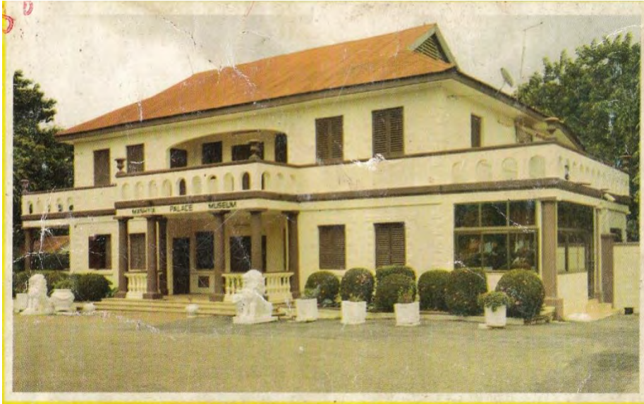
Fig 29. Manhyia Palace Museum, A historic building that exhibit itself.
