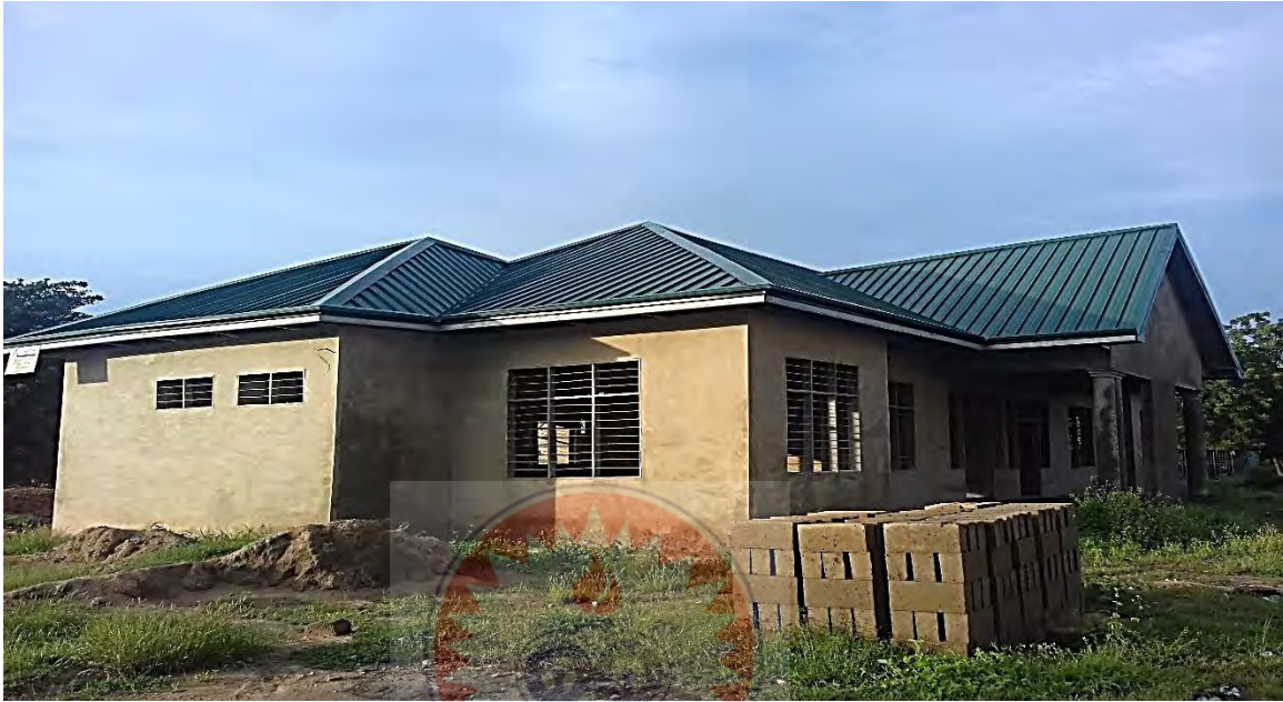
Figure 4.5: ICT laboratory block under construction at Wa Senior High Secondary School.
