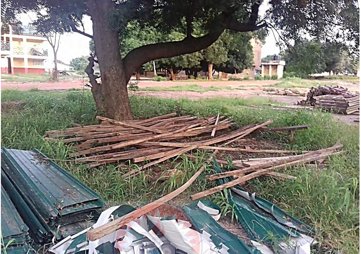
Figure 4.6: Building materials left exposed to the sun and rain at Wa Senior High Secondary School.
