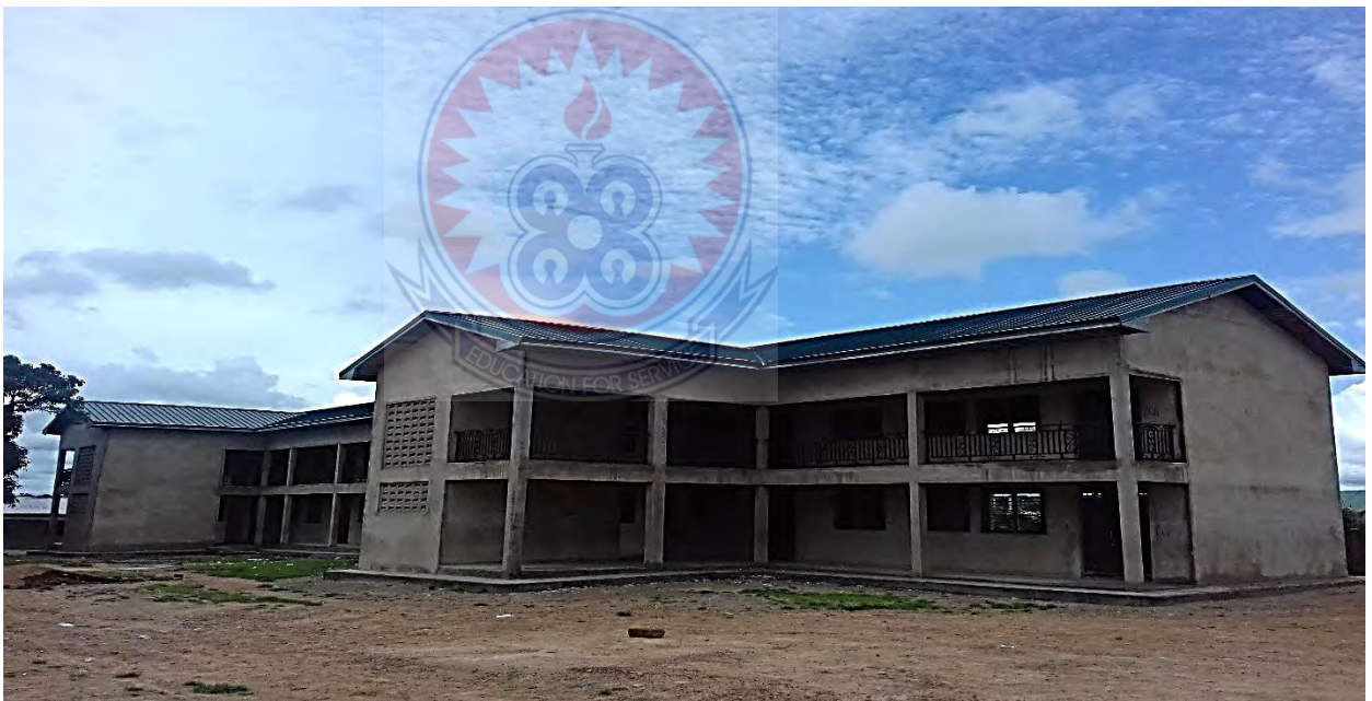
Figure 4.3: 12-Unit Two-Storey classroom block under construction at Fallahia JHS
