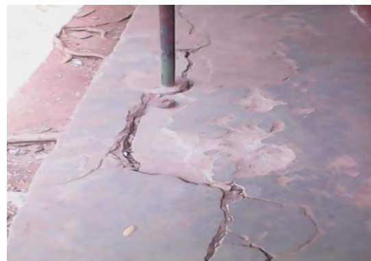
Figure 4. 7 faded and peeled off paints at Charia Primary school
