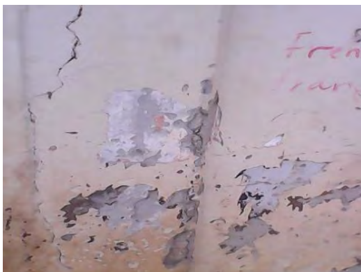
Figure 4.8: crack in floors of the Primary School at Charia
