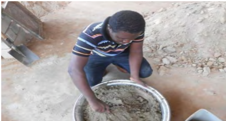
Plate 7: Mixing of mortar
