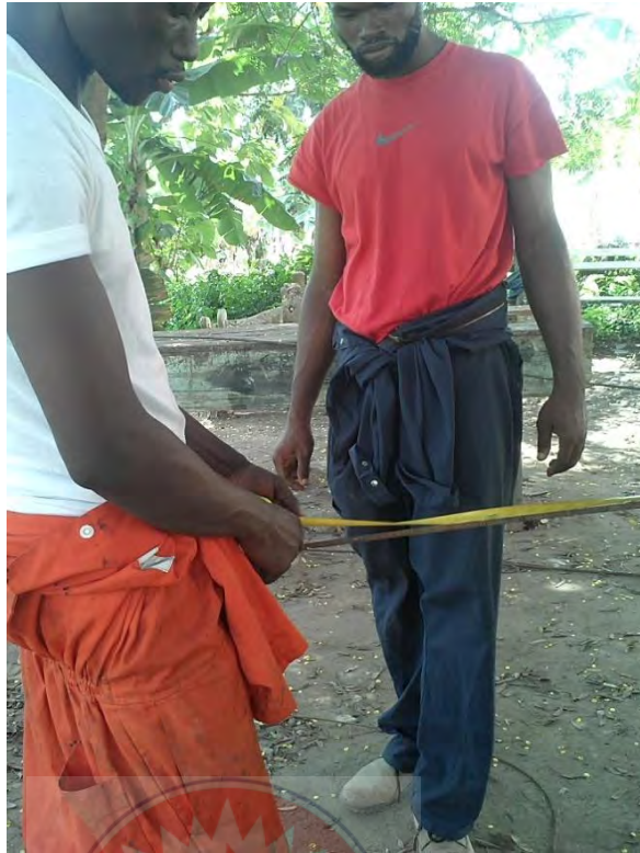
Figure 5.11(B): Measuring of iron rods
