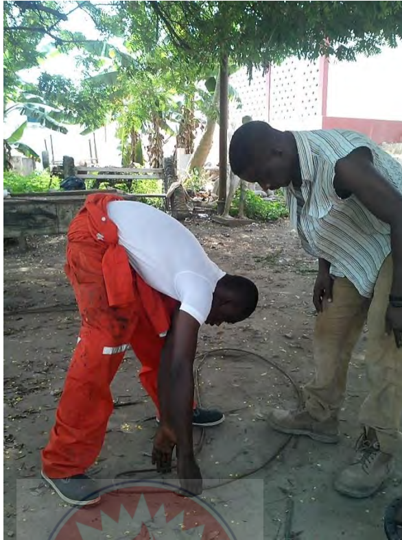
Figure 5.11(D): Bending of iron rod
