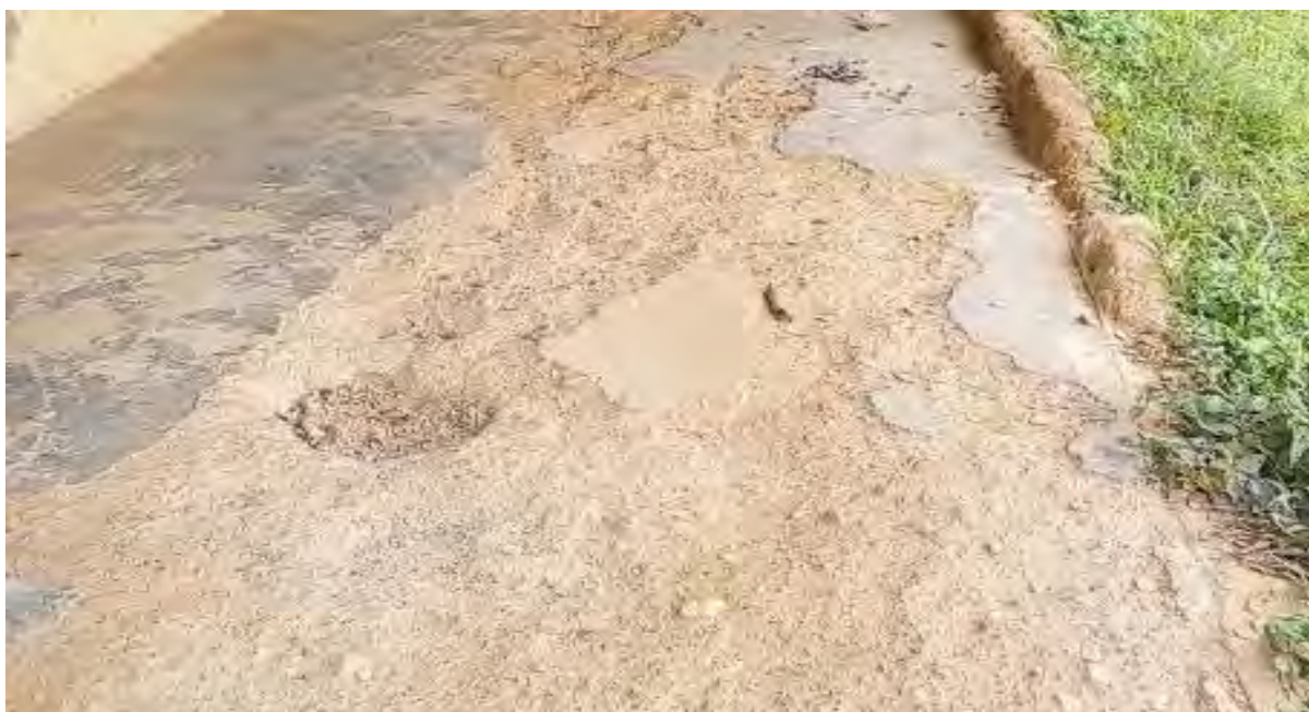
Figure 4.24 Peeled off screed and wearing off floor at Addaekrom D/A Basic School
