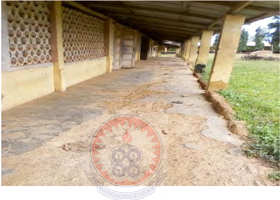
Figure 4.19 Wearing off floor at Takrowase R/C Basic School
