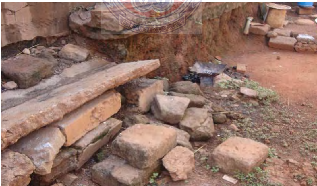
Figure 4. 1 Foundation exposed on buildings of policy makers at Tamale.
