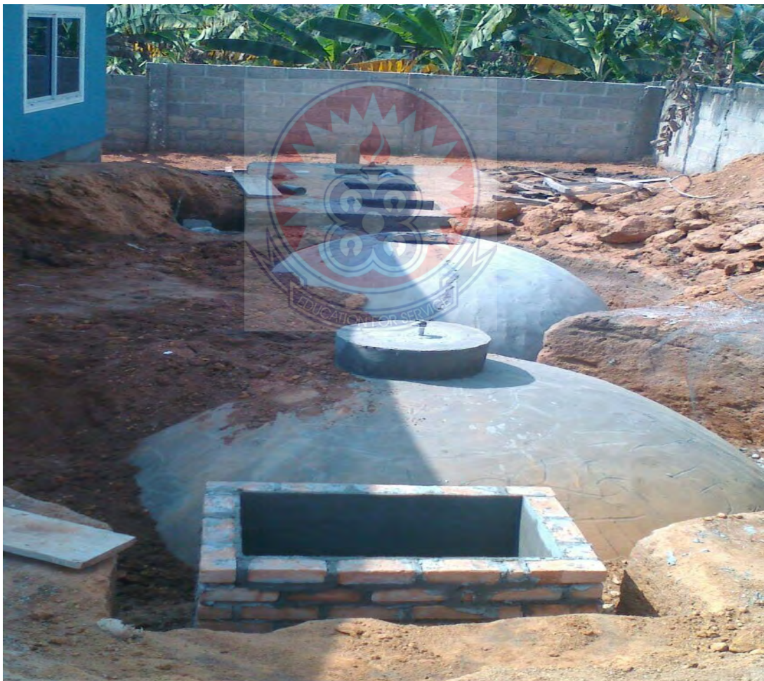
Figure 2.2: Construction of Biogas plant (Wasaza plant)
