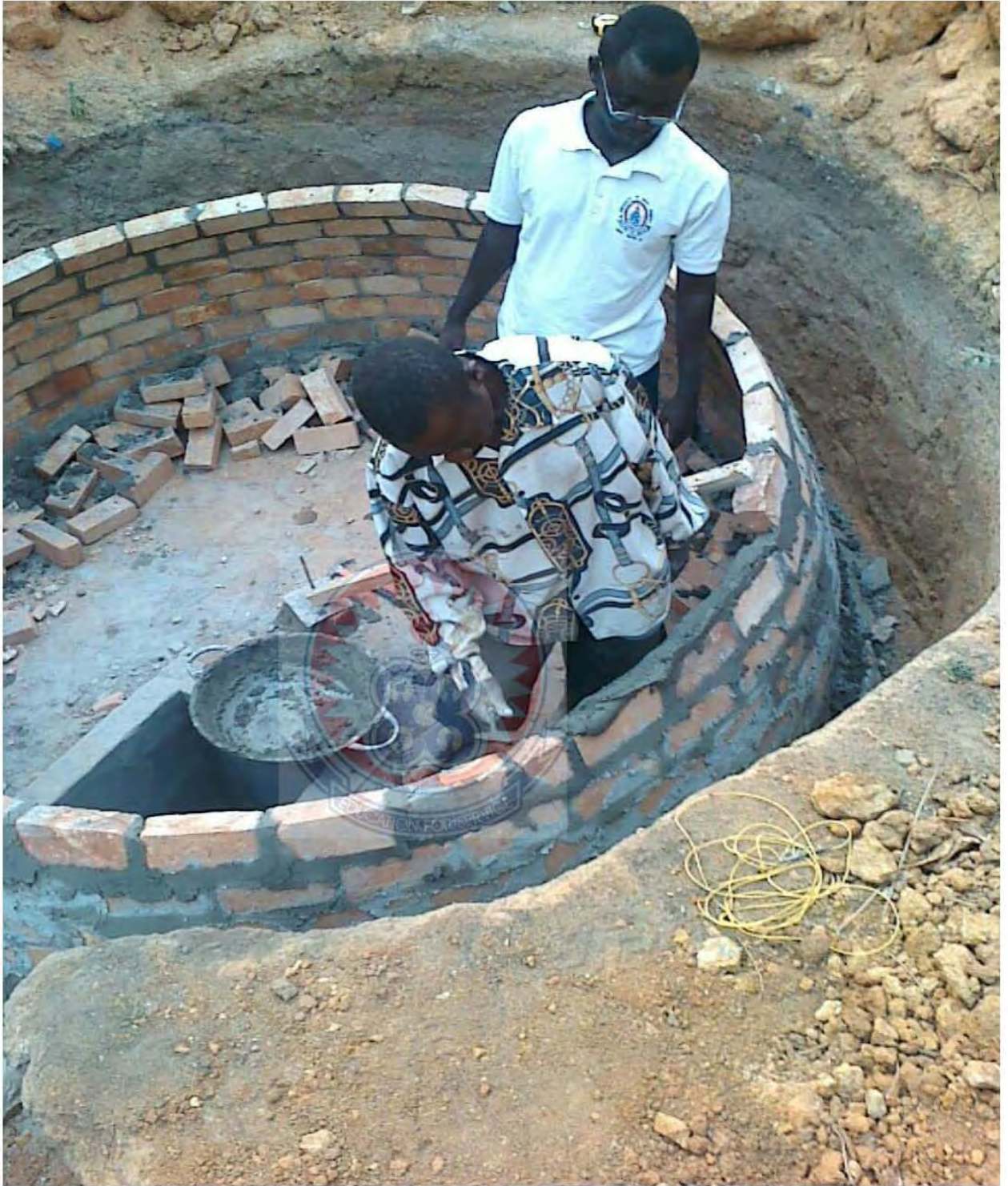
Masons laying bricks
