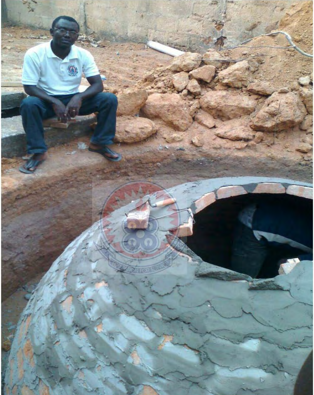
Plastering of the plant
