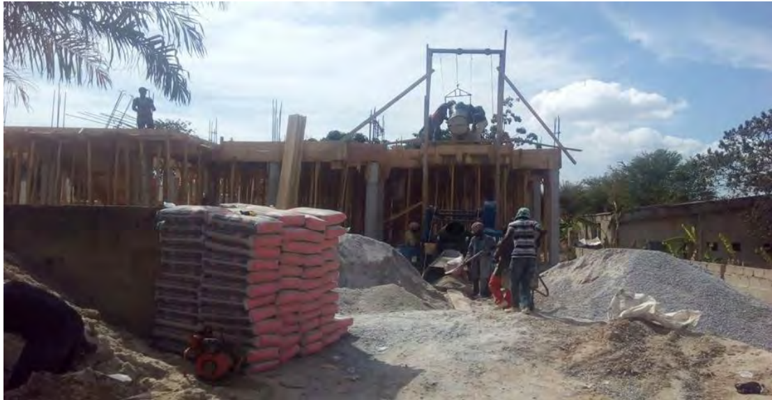
Fig. 4.5: Construction site at Pakoso where construction work was in progress.
