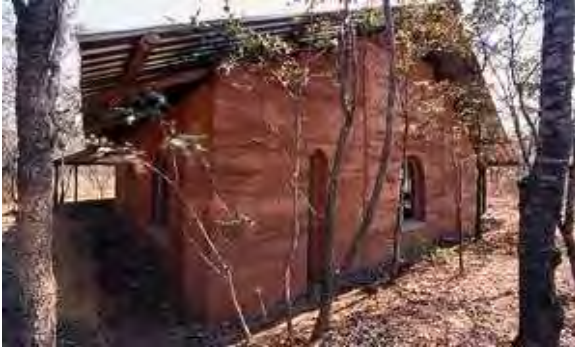
Figure 2.3: Rammed Earth DFID Block at SIRDC, Hatcliffe, Zimbabwe. Source: (Zami and Lee, 2007).
