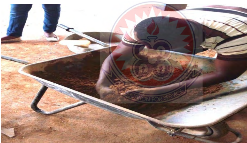
Figure 3.19 Mixing of Soil and Stabiliser
