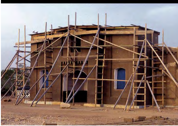
Figure 2.6: Navrongo Basilica Under Construction with Mud
