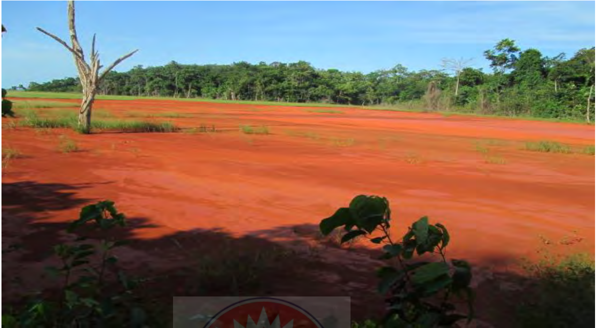
Plate (iii): shows the Terrace Dam Ghana Bauxite Company-Awaso.
