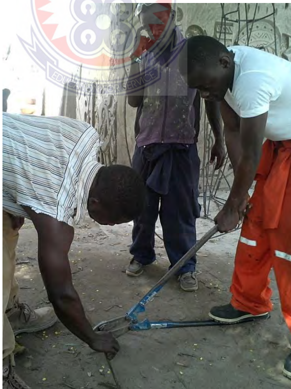
Figure 5.11(C): Cutting of iron rods
