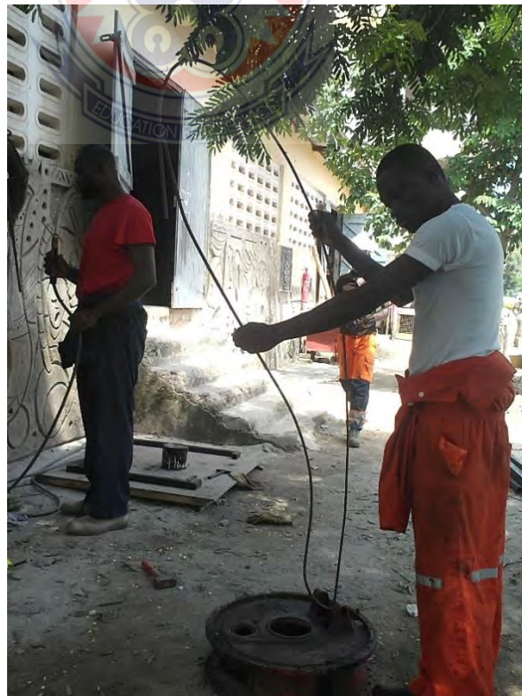
Figure 5.11(E): Testing of bent iron rod on work base
