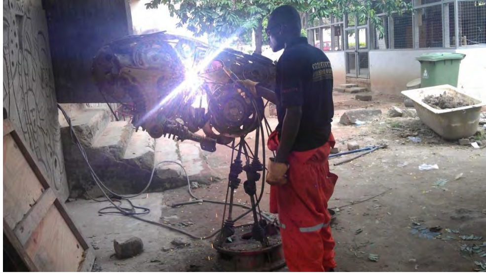
Figure 5.12(A): Arc welding processes of scrap metals into composition.
