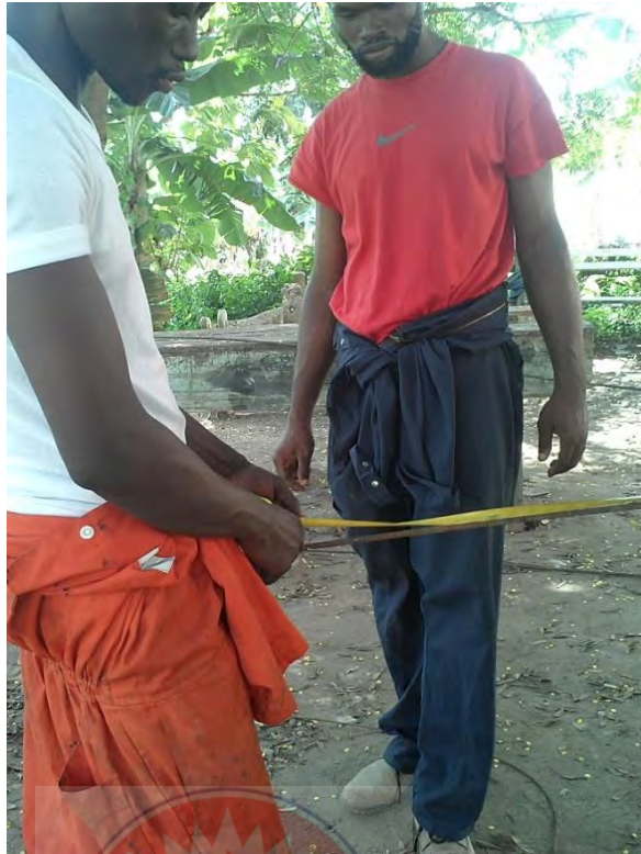
Figure 5.11(B): Measuring of iron rods
