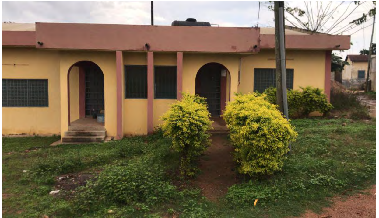
Figure 10: A Renovated Community Library by AYD
