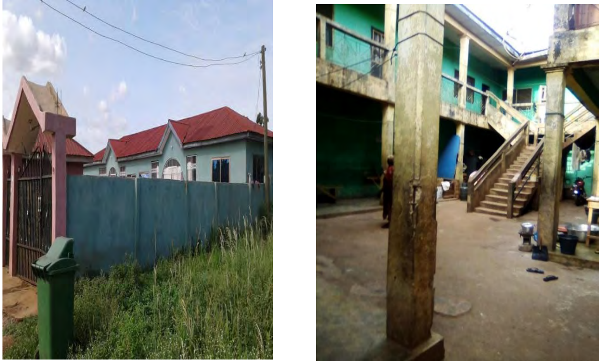
Figure 5: Detached and single storey compound houses in Akrobi
