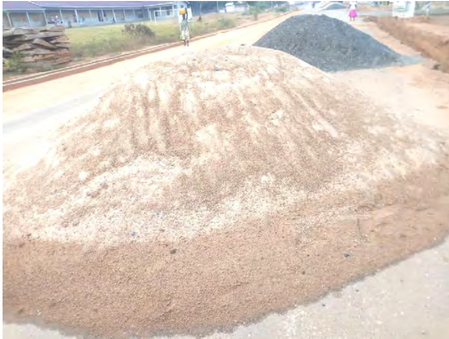
Fig 4.1 shows bally stored aggregates along easting corridor road –Have Afadzato South
