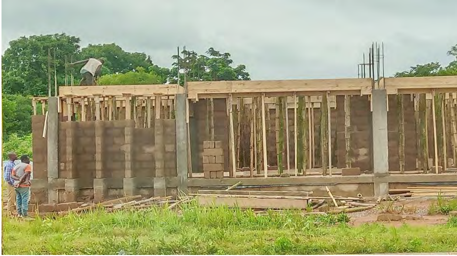
Ongoing construction at Bamahu in the Wa municipality
