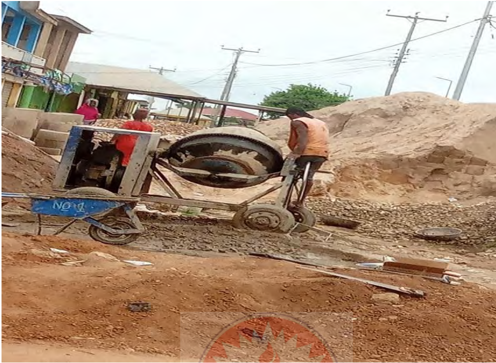
Figure 4.2: Observation at Wa-Sombo where the operator of the concrete mixing machine can slip and fall since he is not wearing wellington boot and helmet.
