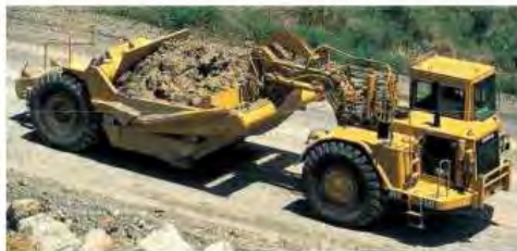
Hauling excavated soil
