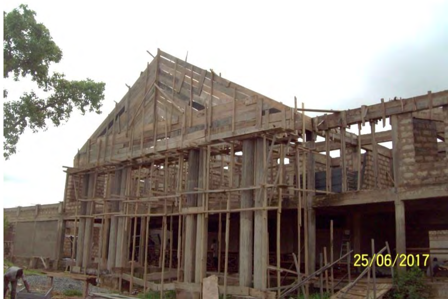
Fig 4.2 scaffold constructed for formwork without guard rails and sole plates at N.J.A College of Education-Wa
