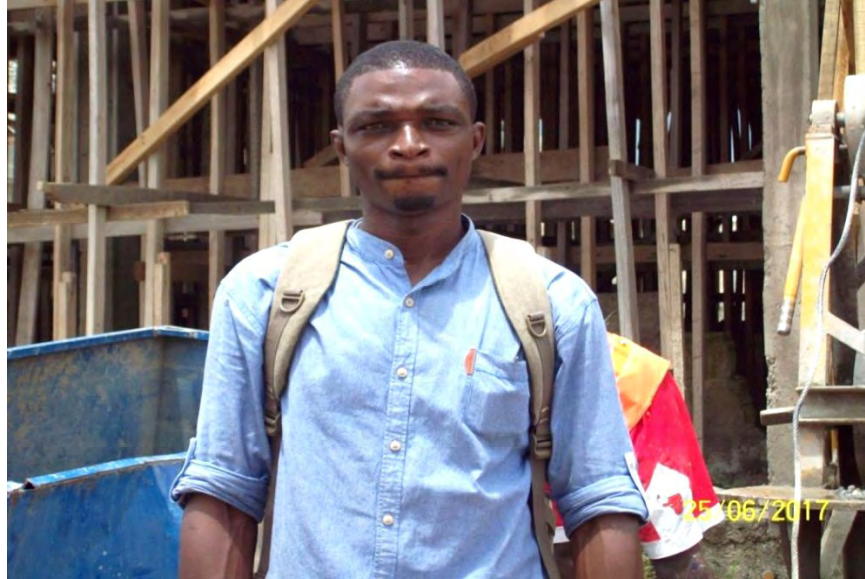
Fig 4.9 As observed props used without sole plates to prevent movement and easy easing of formwork
