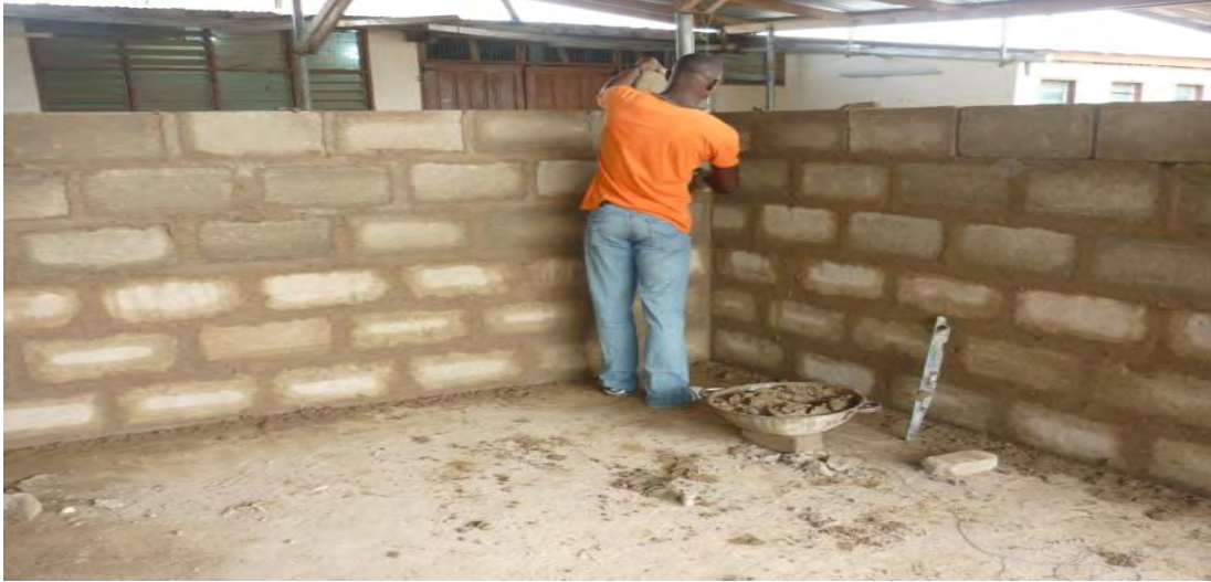
Fig 3.2: Sandcrete block wall
