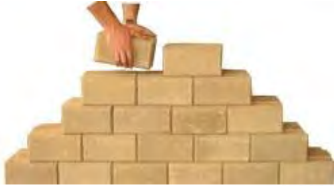
Fig 1: Interlocking blocks being arranged by the craftman
