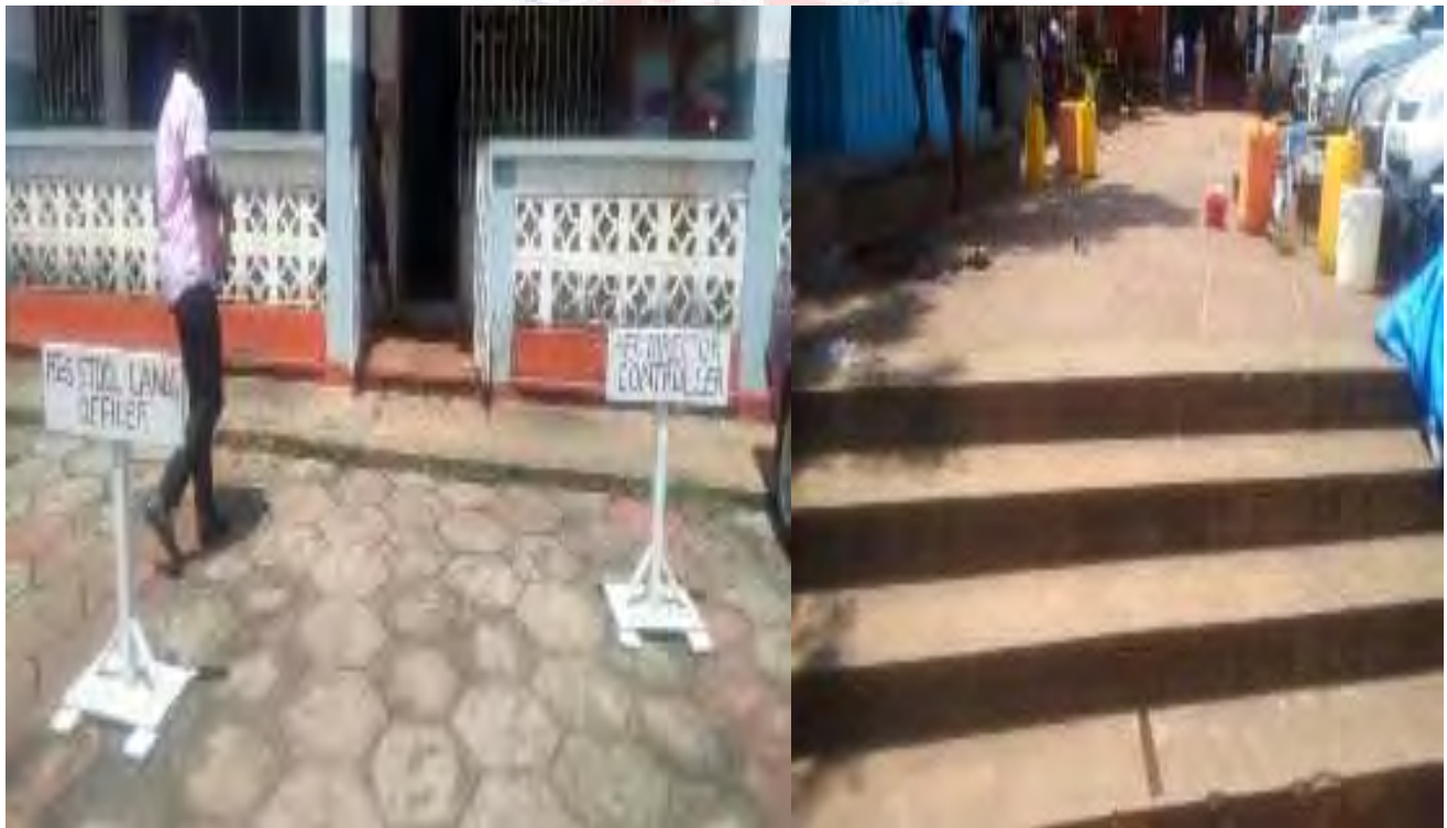
Fig 4.17: Entrances to the buildings at the Kumasi ministries lacks provisions for per persons with disability (Source: field survey 2018)
