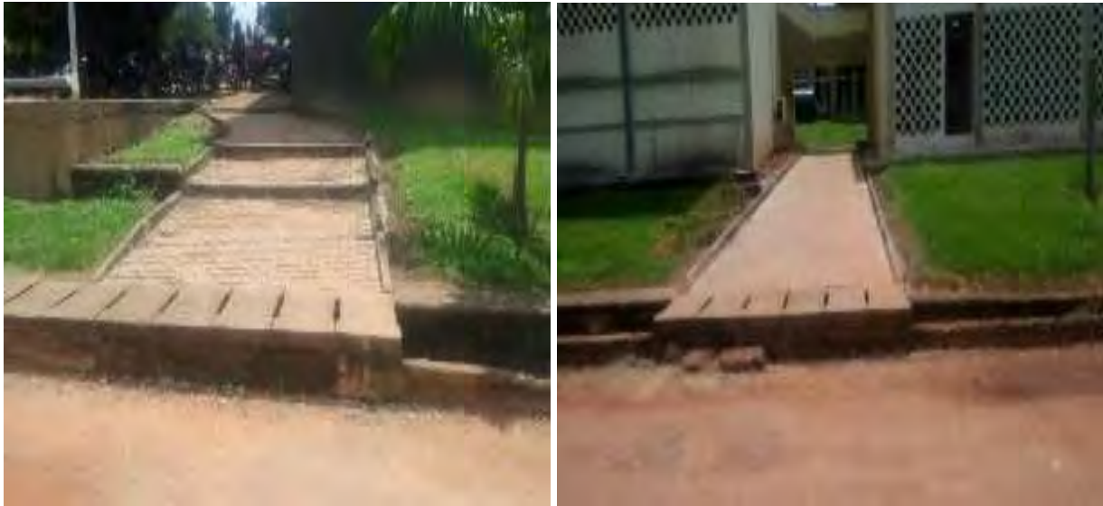
Fig 4.22: There is no provision for Persons with disability to Access the entrance at the Opoku Ware Hall at the UEW- Kumasi (Source: field survey 2018)
