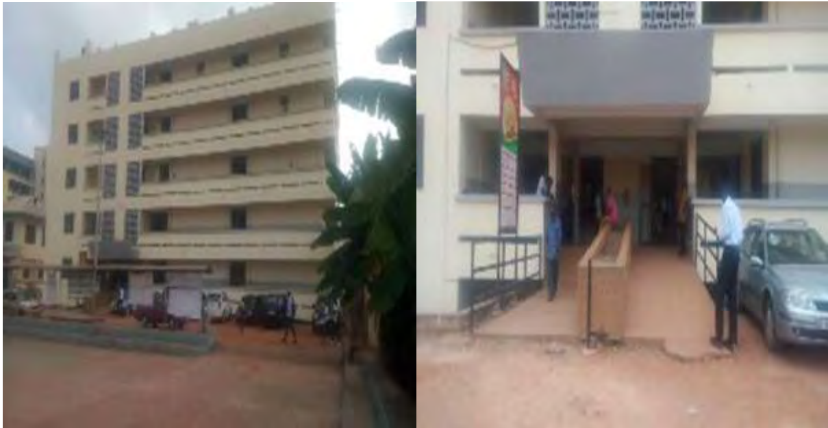
Fig 4.35: The newly constructed MP Block at KsTU, Kumasi has guarded ramp at the entrance but lack those provisions at other parts of the building. (Source: field survey 2018)
