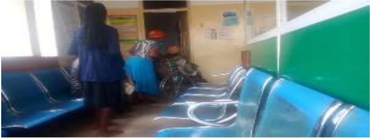
Fig 4.12: Entrance to consulting rooms in Sunteso hospital lack adequate ramp at the entrance. (Source: field survey 2018)
