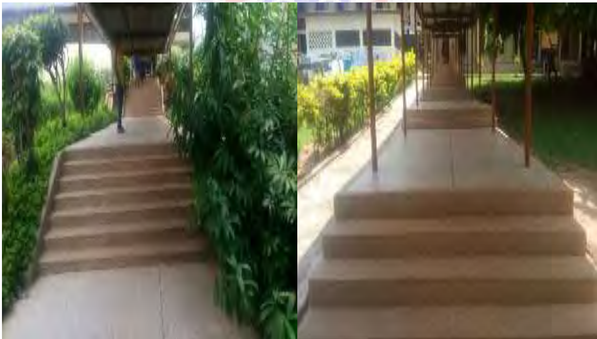
Fig 4.21: These walkways at institutions UEW- Kumasi are not friendly to the disable. (Source: field survey 2018)
