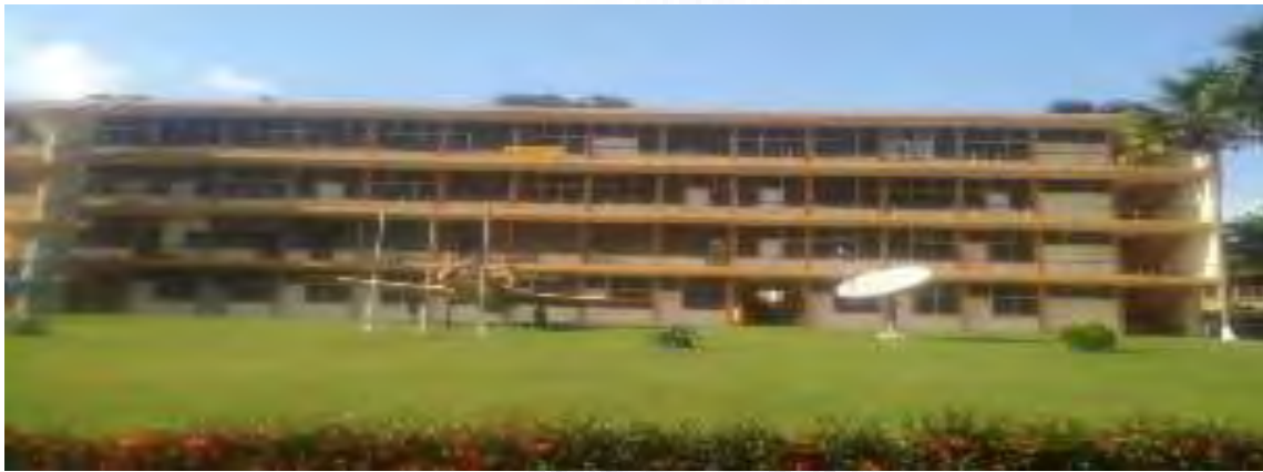
Fig 4.28: College of Engineering building at KNUST, Kumasi Lacks provisions for both horizontal and vertical movement for the disabled . (Source: field survey 2018)
