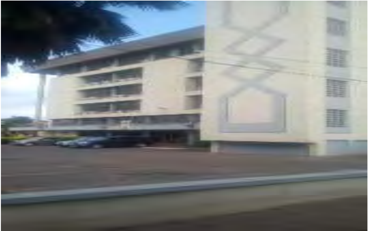
Fig 4.32: The main administration block At KsTU, Kumasi has elevator but lacks provisions for the disable at the entrance and inside the auditorium.
