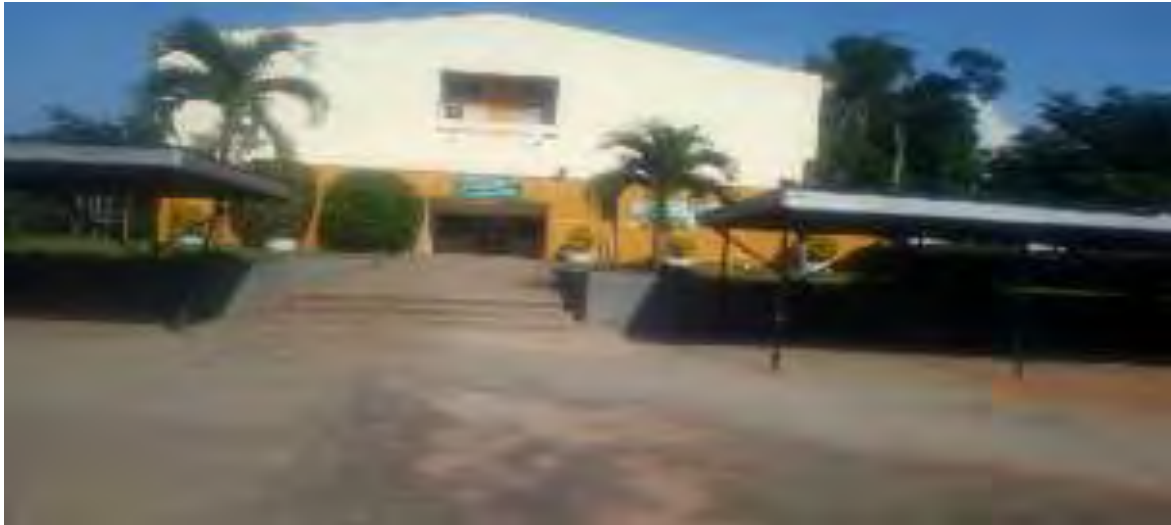
Fig 4.31: Center for drug analysis quality control Kumasi lacks provisions for the disabled at the main entrance. (Source: field survey 2018)
