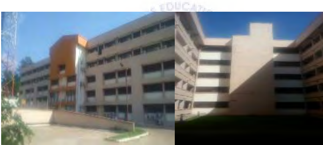
Fig 4.30 Institute of Distance Learning (IDL) building Lacks provisions for both horizontal and vertical movement for the disabled KNUST, Kumasi. (Source: field survey 2018)
