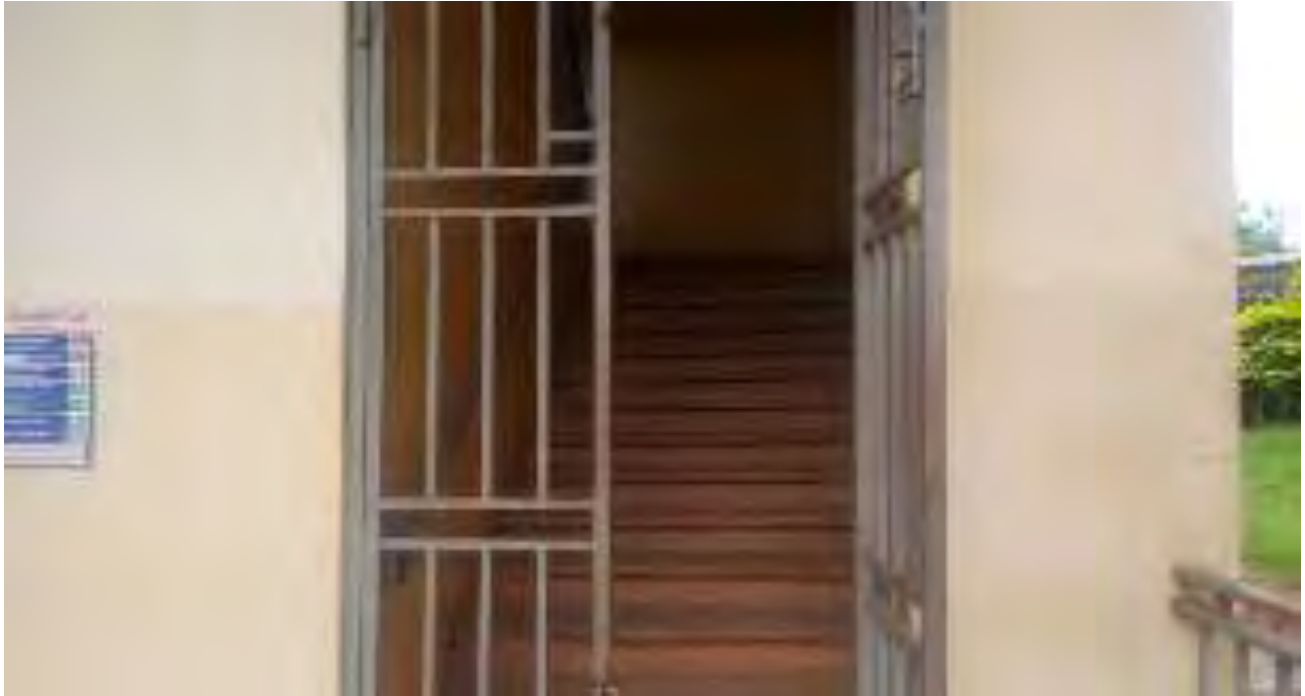
Fig 4.19: The Library, Computer lab and lecture block of the EUW, Kumasi lacks provisions for vertical and are only accessible through stair. (Source: field survey 2018)
