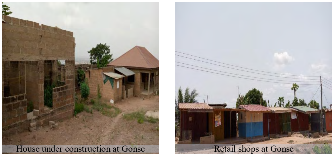
Figure 15: A section of house under construction and retail shops at Gonse
