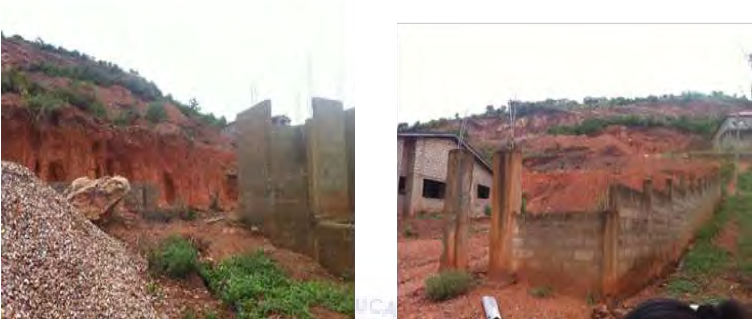
Plate 4.2: On-going construction works at the taxi rank area
