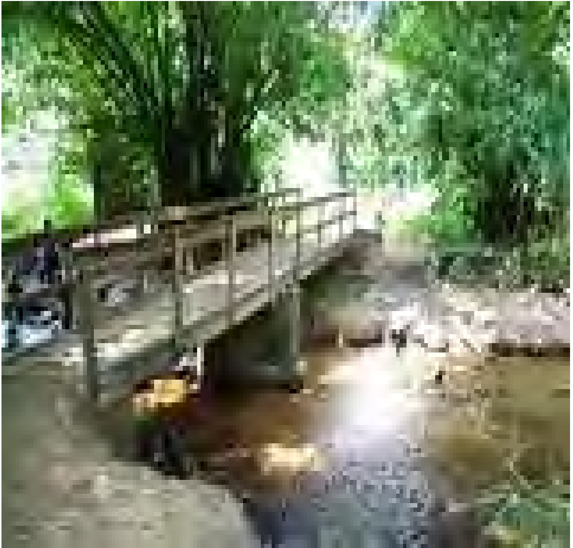
Fig.3.4. The first foot Bridge at the entrance into the Agumatsa Wild Life Sanctuary
