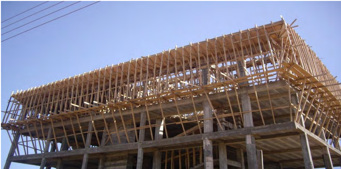
Plate 7. Timber Formwork for a Storey Building Source: New Officer Block (Burma Camp), Accra.
