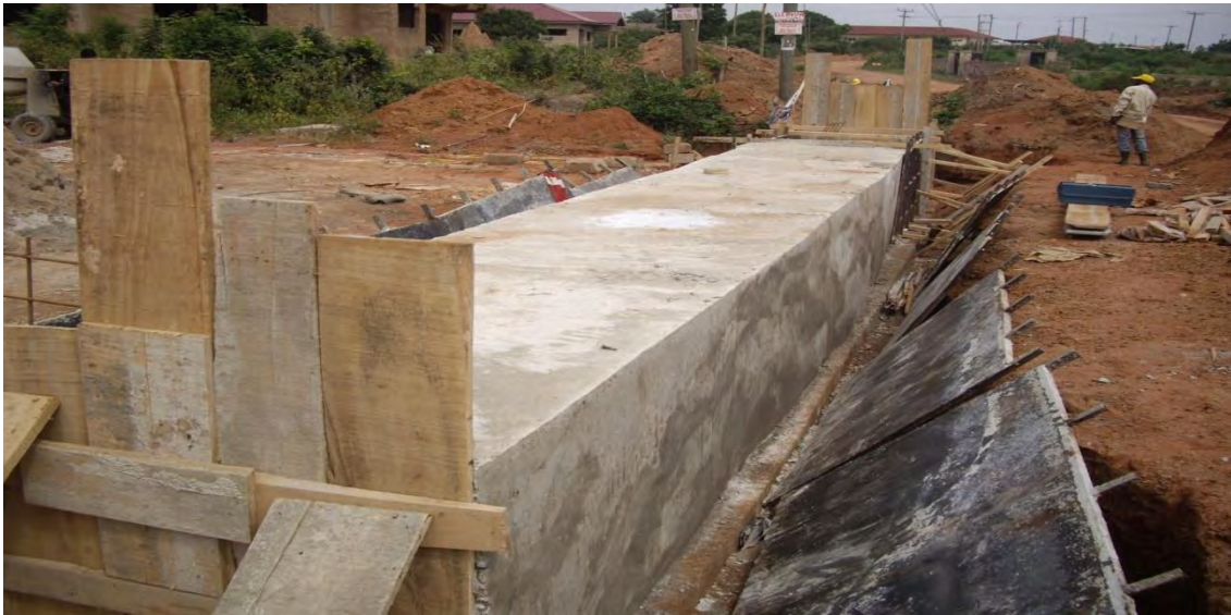
Plate 9. Timber Formwork for Reinforced Concrete Culvert Source: Giffard Road, Burma Camp, Accra. China State Haulong
