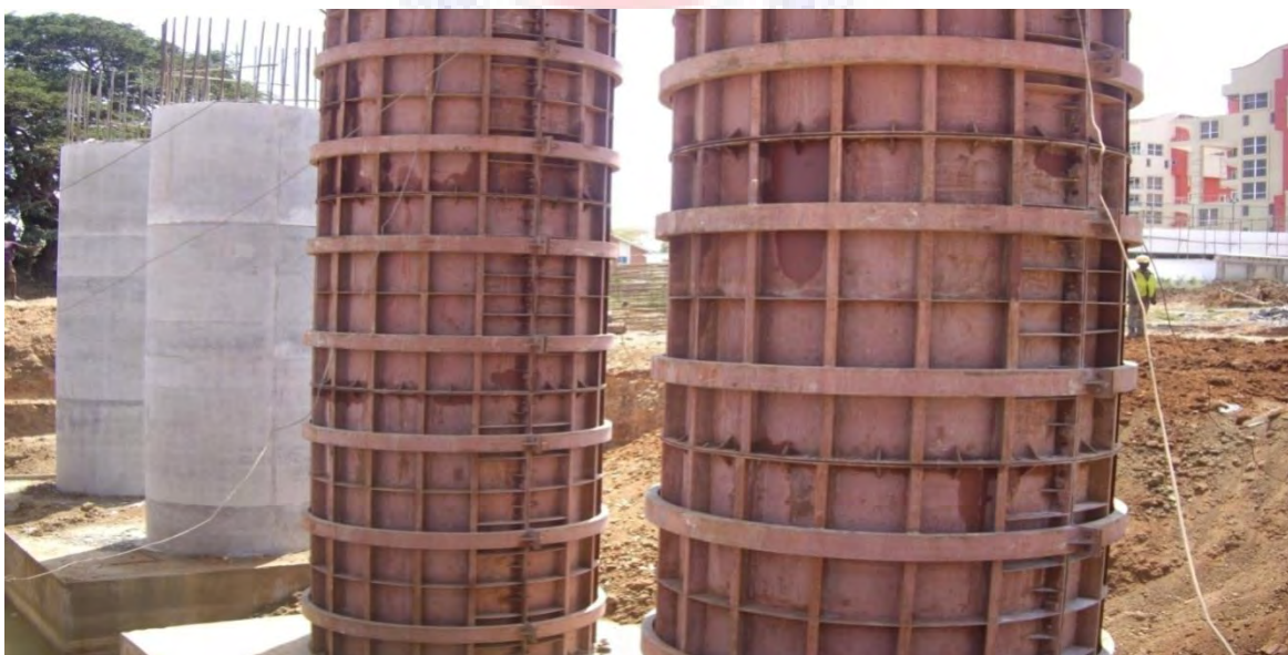
Plate 14. Erected Circular Column Steel Formwork Source: Source: Giffard Road, Burma Camp, China State Haulong
