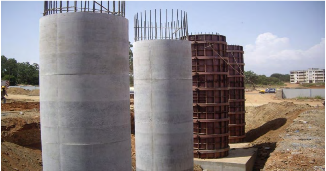
Plate 15. Reinforced Concrete Circular Column after Striking Source: Source: Giffard Road, Burma Camp, China State Haulong
