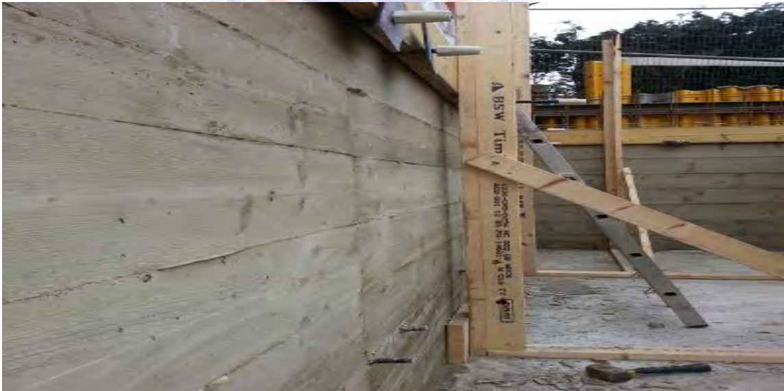
Plate 10. Poor Concrete Finish of a Timber Formwork. Source: Source: Giffard Road, Burma Camp, Accra. China State Haulong
