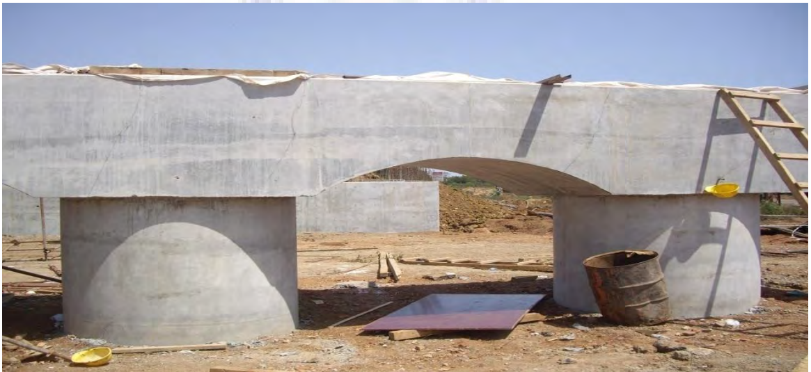
Plate 16. Reinforced Concrete Structure after Using Steel Formwork Source: Source: Giffard Road, Burma Camp, China State Haulong
