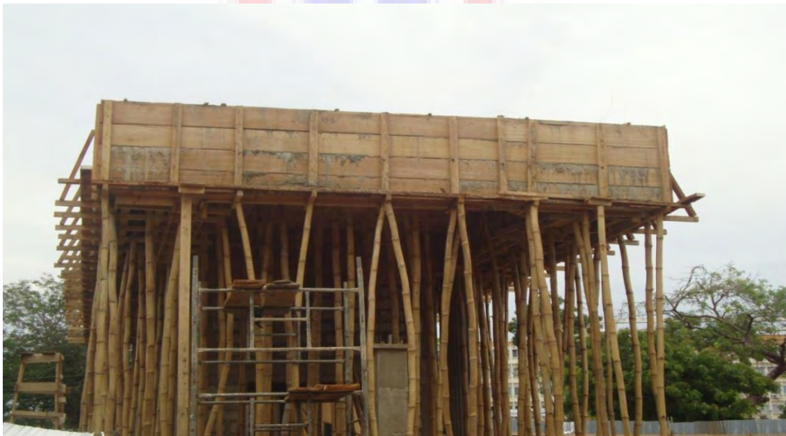
Plate 7. Timber Formwork for a Storey Building Source: New Officer Block (Burma Camp), Accra.
