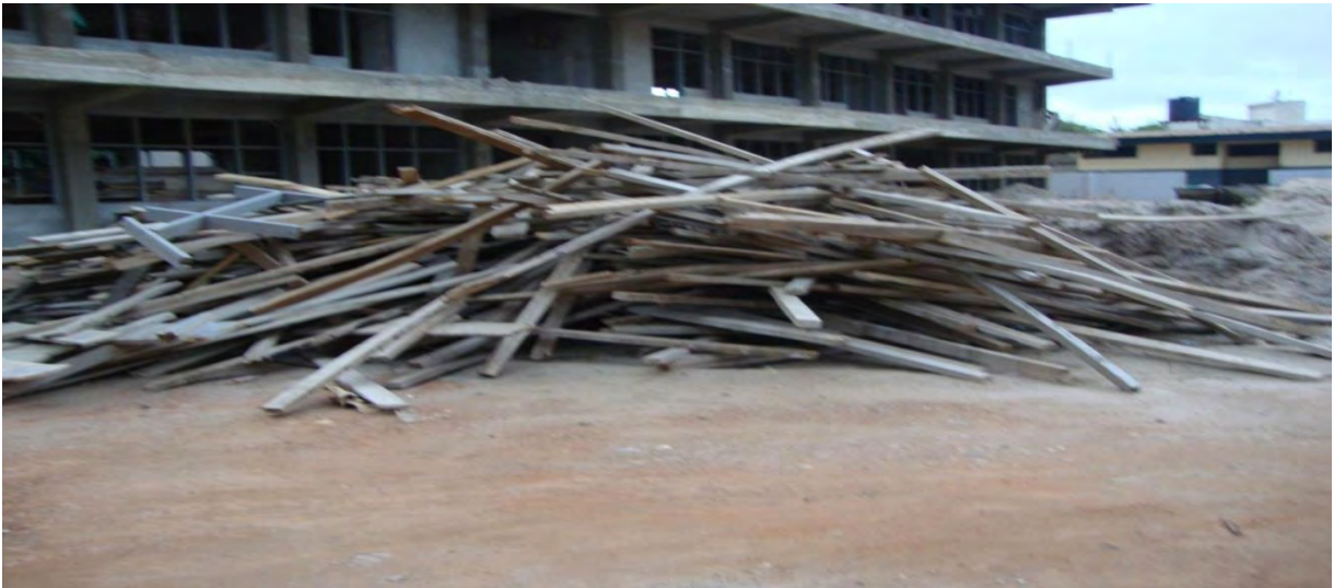
Plate 11. Poor Stacking of Timber Removal. Source: Kinbu Sec. Tech. School (New Class Room Block), Accra.
