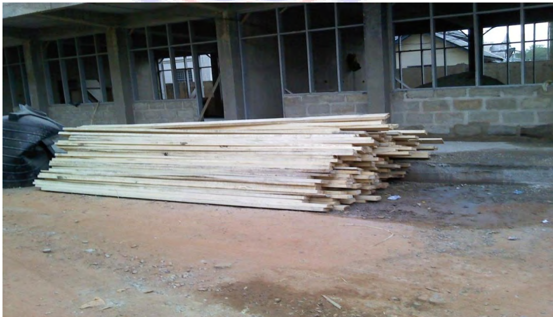
Plate 6. Poorly Stacked Fresh Timber at a Site Source: Kinbu Sec. Tech. School, Accra (New Class Room Block).
