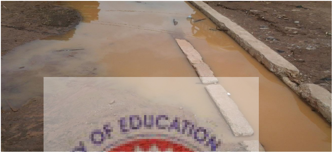
Plate 4.9: Flooded gutter
