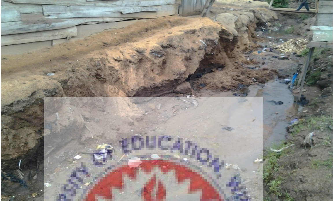
Plate 4.11: Sawdust closing drainage
