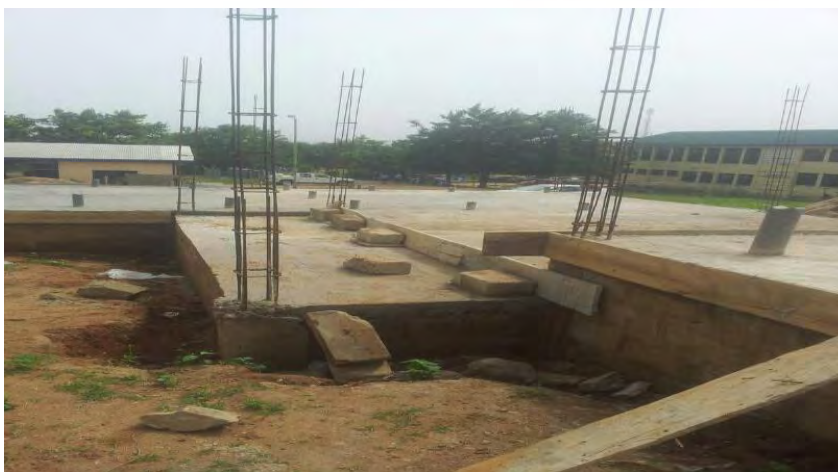
Figure 4.6: 6 unit classroom Koforidua Technical Institute
