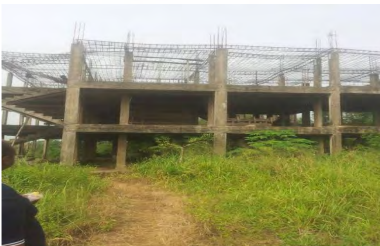
Figure 4.9: Affordable House in Koforidua
