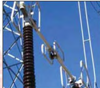
Figure 8: Disconnect Switch
