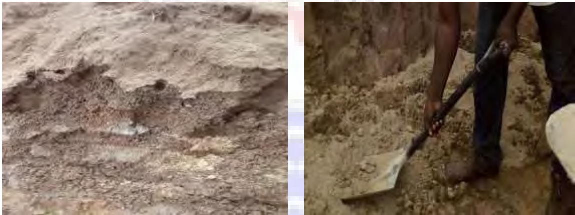
Figure 4.2: Sand for manufacturing of OPC and pozzomix cement sandcrete blocks and the batching and mixing processes at Aprade construction site.
