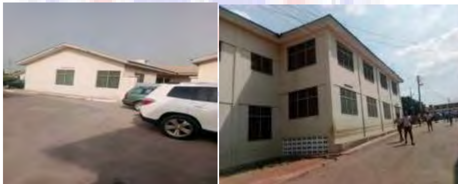
Other existing structures at Anglican SHS constructed with OPC sandcrete blocks
