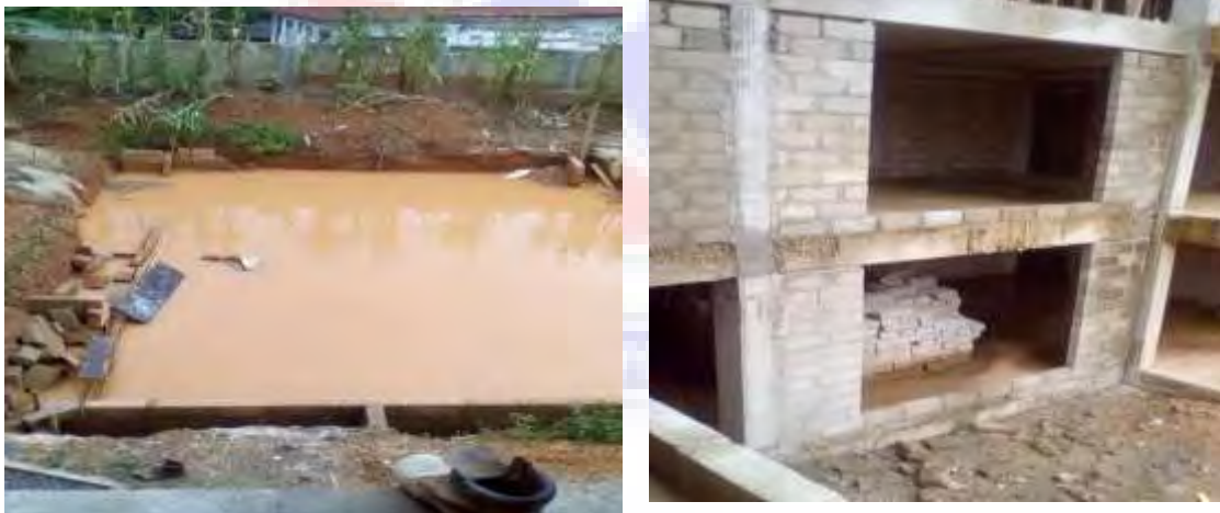
Figure 4.5: Construction of hotel complex in a water-logged area at Danyame, Kumasi
