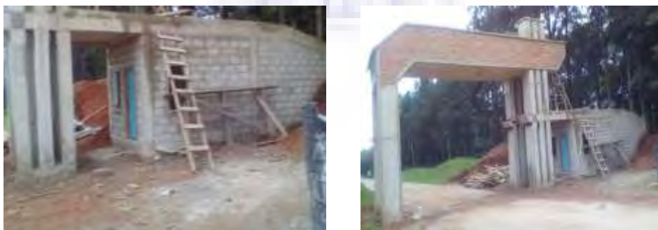
Figure 4.4: The newly constructed entrance of CSIR-BRRI at Fumesua near Kumasi with pozzomix cement sandcrete blocks. Source: Researcher Field Construct, 2018
