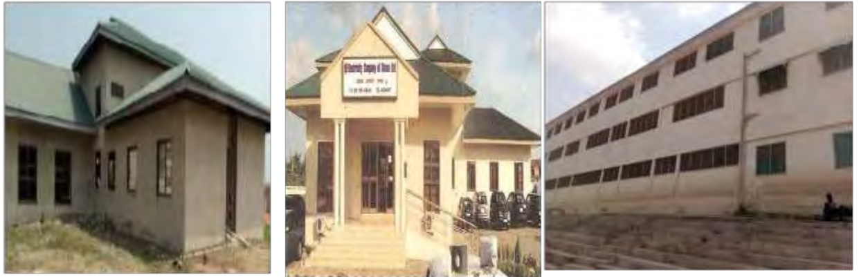
Figure 4.3: Pozzomix cement sandcrete blocks office complex for ECG and Dormitory Block for Kumasi Anglican SHS Researcher Field Construct, 2018
