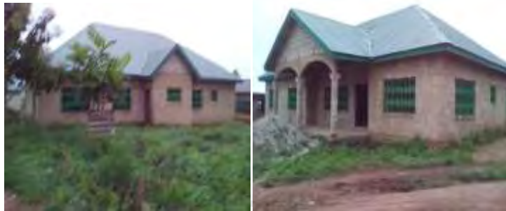
A residential structure under construction with pozzomix cement at Fumesua
